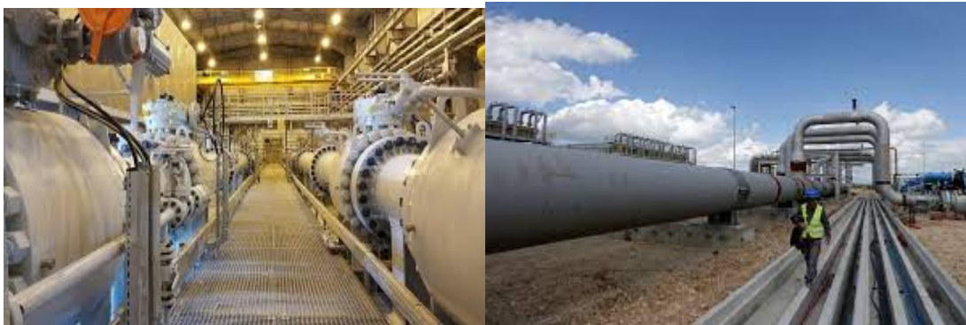
Figura 108 TAP pipeline exit point in Fier
