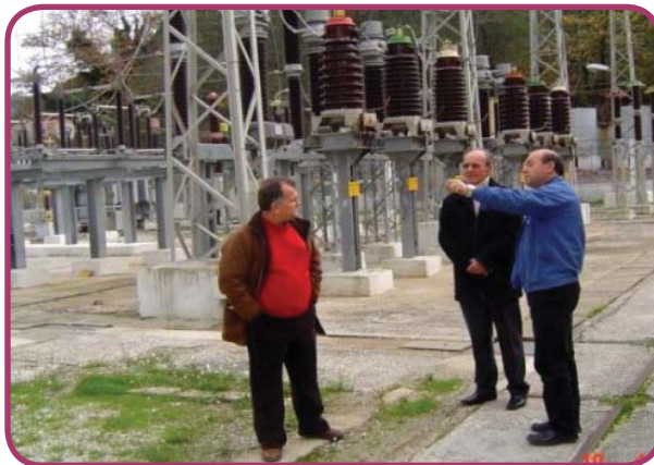
Site visit in Bistrica HPP after construction. Bistrica, 11th December
